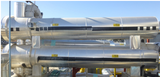
Figure 1. Shell-and-tube heat exchanger
