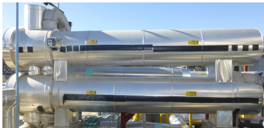
Figure 1. Shell-and-tube heat exchanger
